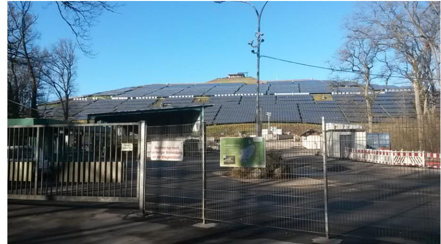
Solar array on the local landfill – Freiburg
