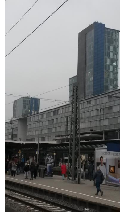
More solar panels on high rise building in Freiburg
