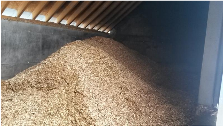
Wood chips for district heating scheme supplied by local foresters
