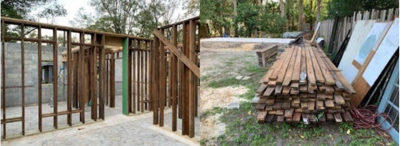
Figure 12 Reclaimed timber framing. Photos, Bradley Guy.
