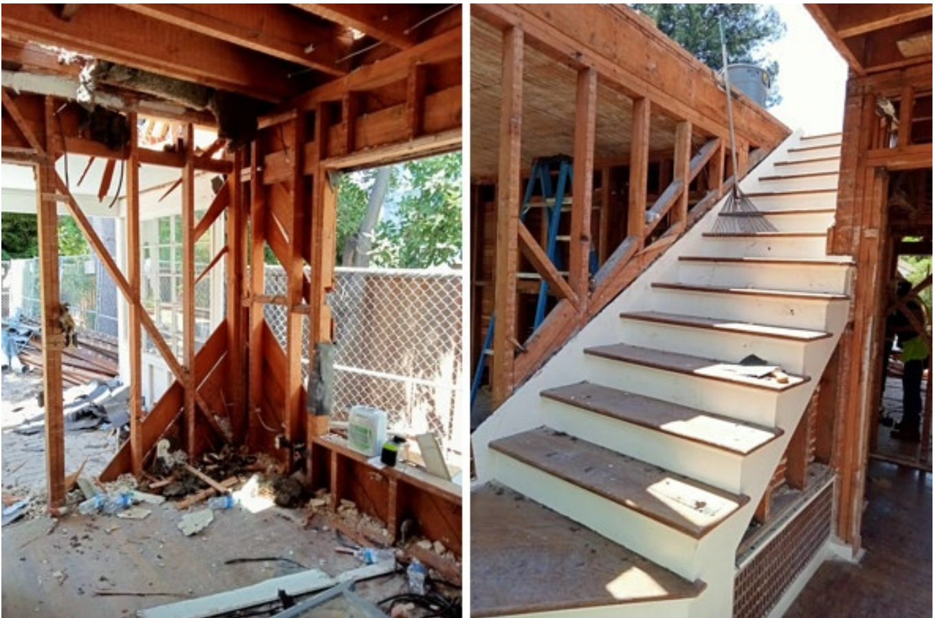
Figure 17 Residential building undergoing deconstruction in Palo Alto
