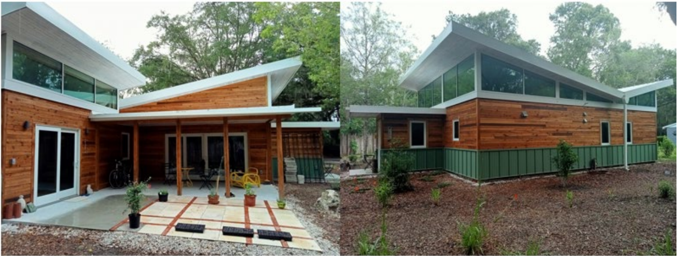
Figure 13 Reused timber can be seen in the cladding and soffits.
