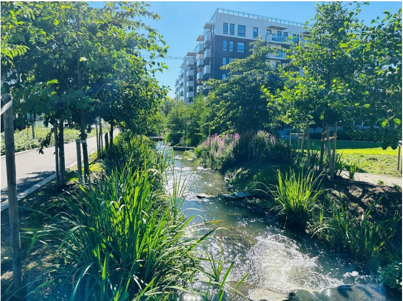
Figure 3: Daylighted stream adjacent to street conveying stormwater diverted from the combined wastewater-stormwater system in Oslo
